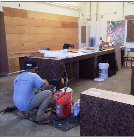
Drake Olaso from Stan's Contracting mixes drywall joint compound in the science lab.
